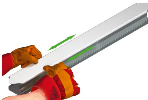
Fig. 4.8: Fitting the beginning of the tape
